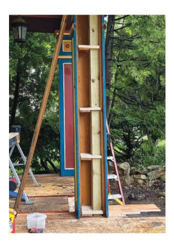
We had to cut back the rafters so they were no longer nailed to the house and wouldn't pinch as we jacked the roof up. With the roof system shored up and everything cut back, we were able to easily use the screw jacks to lift the roof to level. We then cut the rafters back further so we could slide a 2x6 ledger in. We screwed the ledger into the studs and screwed the rafters to it.
